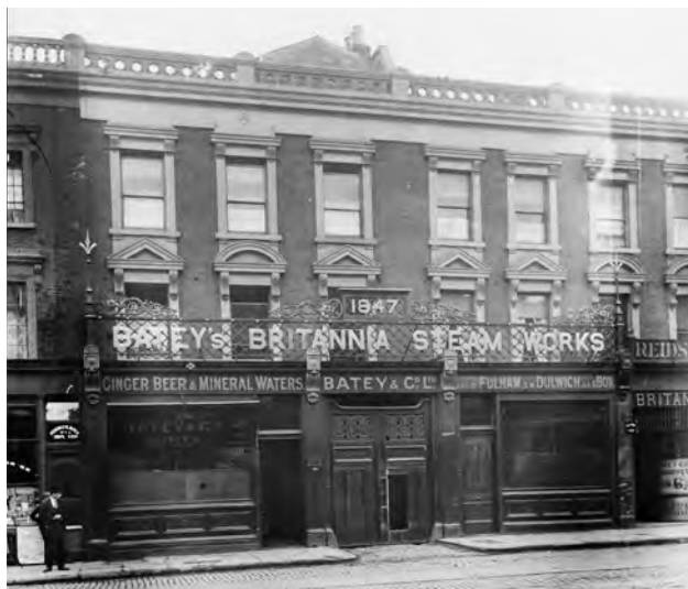
Figure 1: The Kingsland Road frontage to Britannia Steam Works in about 1920 (HA P3597).
