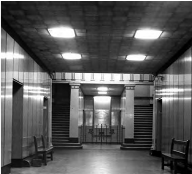
Figure 5: The Entrance before restoration – with boxed-in original detailing and covered floor – 1978: HA P8534
