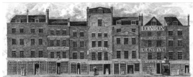
Leadenhall Street 1823: Heather's business is now under the name of J. W. Norrie at 157, second door on the left – though without the 'Little Midshipman'
